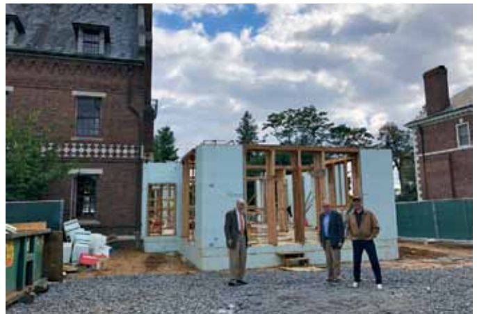
Dennis Keller '63, Tom Fleming '69, and Wistar Wood '83 checking on the progress.
