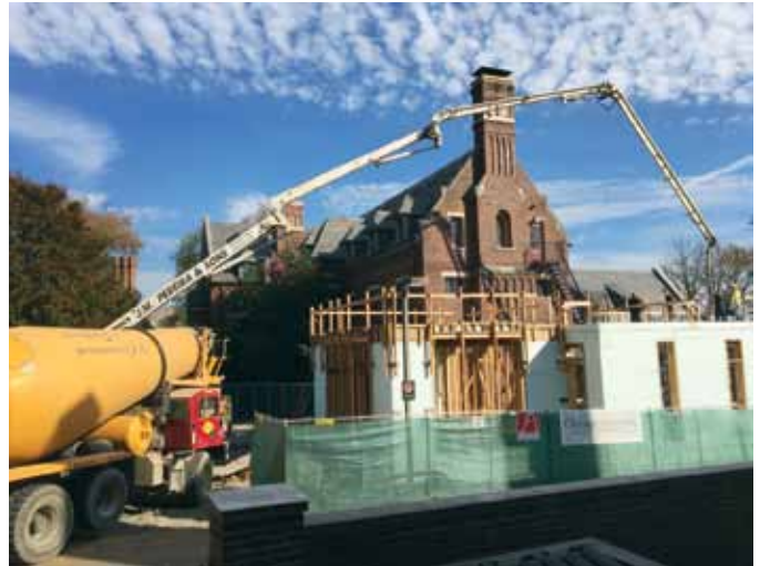
Pouring the concrete for the Cox Wing
